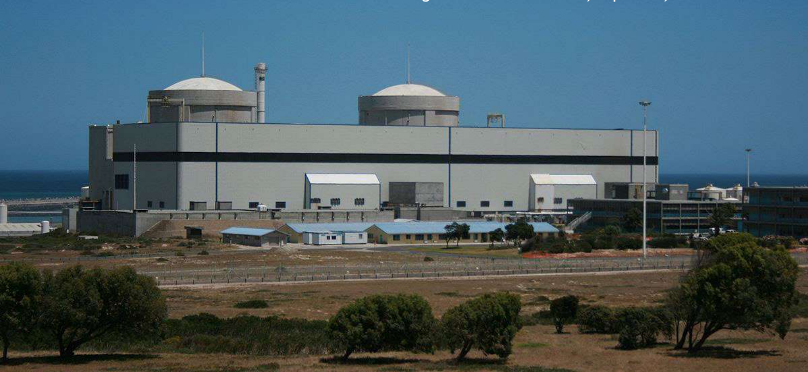
Koeberg Nuclear Power Station, Capetown, South Africa
