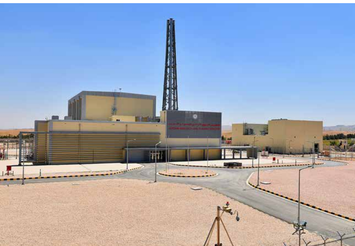
Front view of the Jordan Research & Training Reactor (JRTR) located outside the Jordan University of Science & Technology in Irbid Town north of the capital City of Amman.
